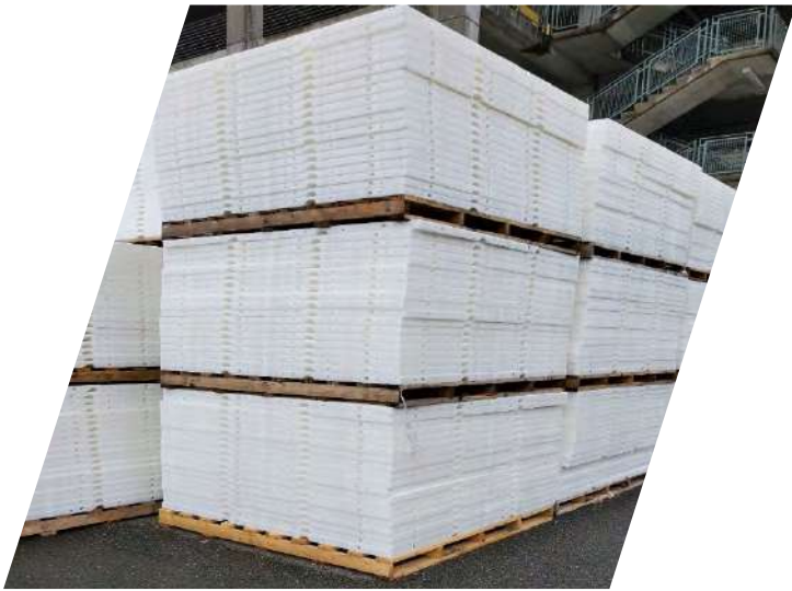
New terraplas-NF tiles stacked and ready to fit
